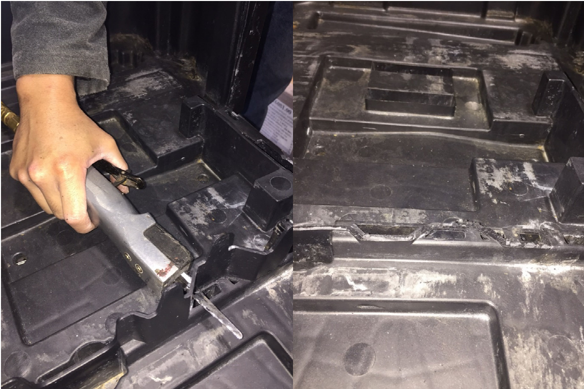
Fig. 6- Raised material removed.
